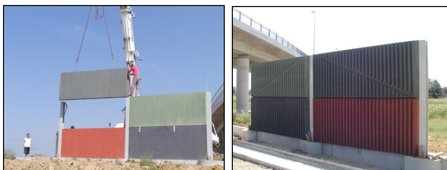
Figure 5 Installation of test section of RUCONBAR panels
