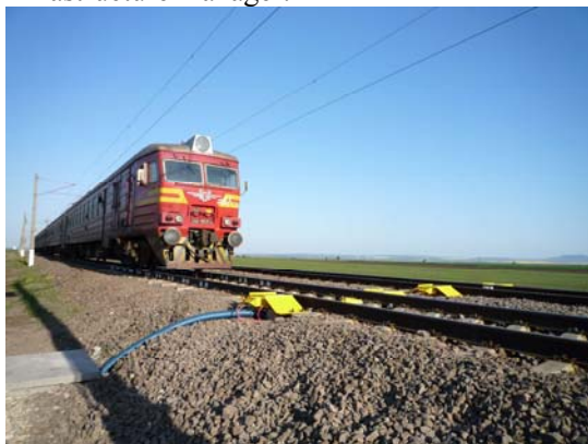
Fig. 3 Test installation at Zimnitsa
